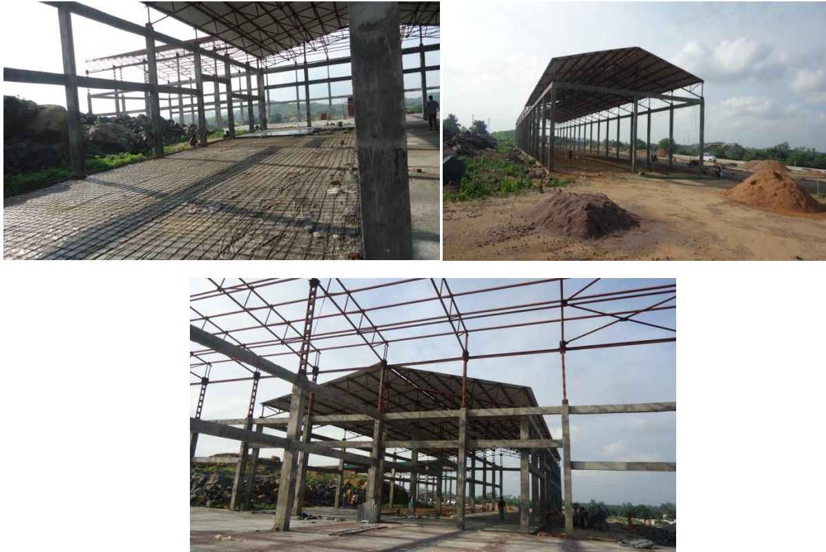
Figure 10: Integrated Solid waste management plant under Construction
